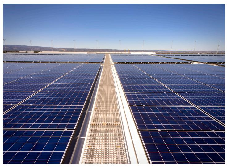
Completed in March 2016, the system has utilised leading edge technology consisting of 4,500 high quality tier 1 TrinaSmart 260W solar panels with DC power optimisation and 18 SMA inverters - thus providing safe and reliable renewable energy of 1,768 MWh.
